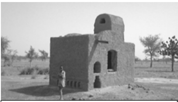
Pottery kiln run by women, built with woodless construction, Burkina Faso
